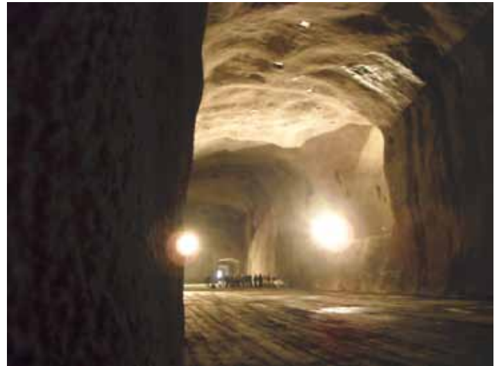
100x20x20 m cavern in the Gonzen near Sargans, where a modern semiconductor foundry is being constructed by Espros Photonics Corporation for the production of high-performance CMOS/CCD image sensor chips made 100% in Switzerland
